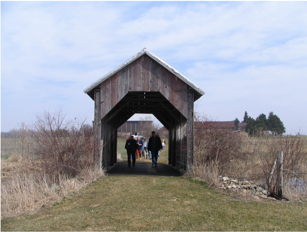
Restored covered bridge on Harry Nelezen property
